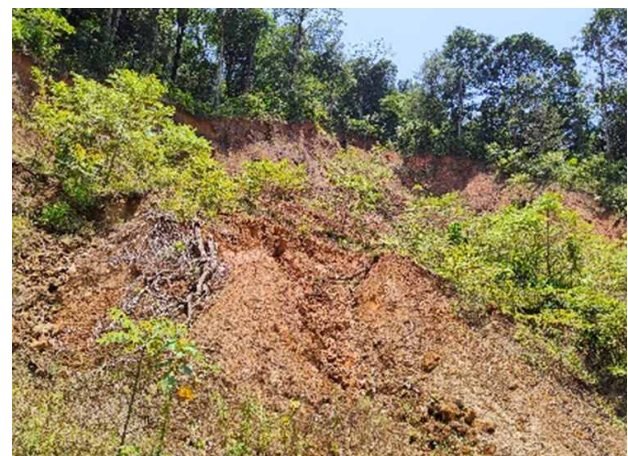
Fig. 2. Naturally vegetated landslide area.
