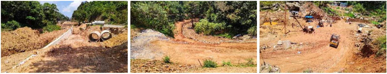
Fig. 4. Rehabilitation tasks in landslide region along the roadsides.
